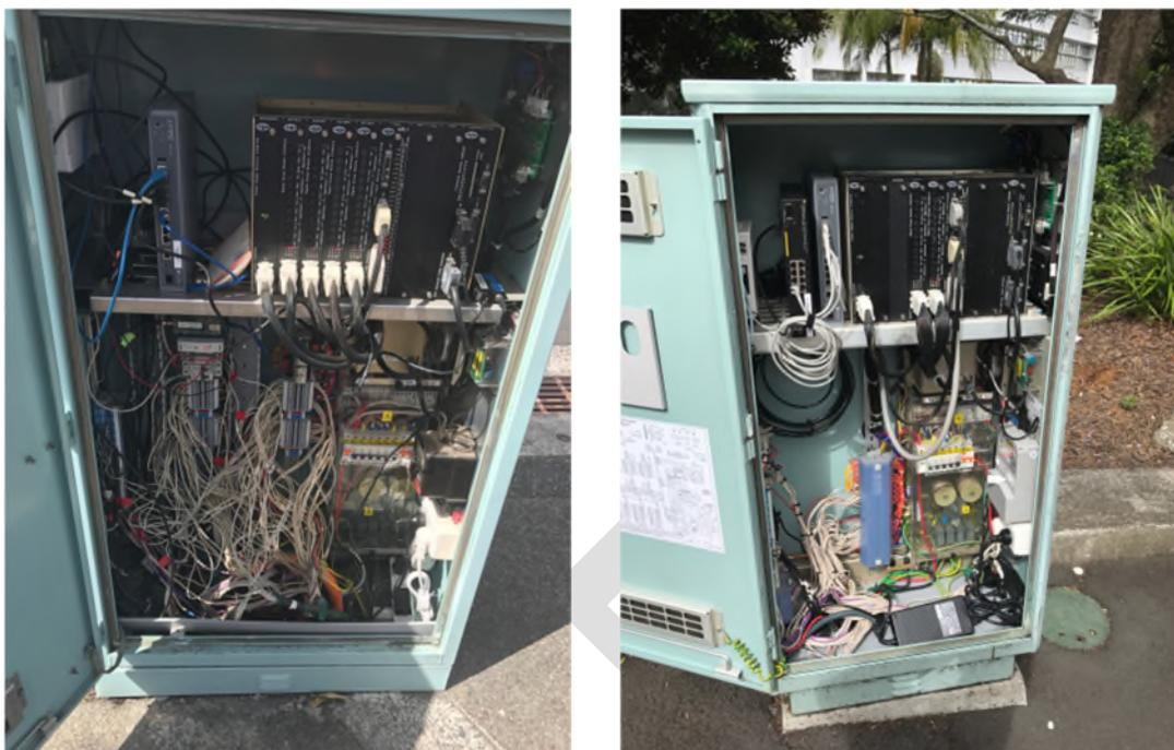
Depending on the existing hardware available at the cabinet, the minimum addition into the cabinet will be a network switch to connect multiple cameras into the network. Uninterruptable Power Supplies could also be considered to provide operation or at minimum a graceful shutdown of systems in case of a power failure.
