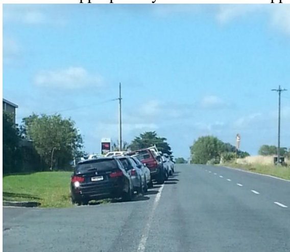
Fig 5 Example of significant safety hazard due to lack of parking On Postman Road outside airfield office
