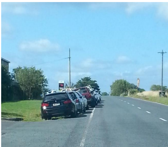
Fig 5 Example of significant safety hazard due to lack of parking
