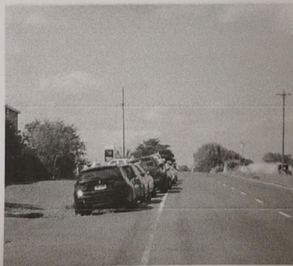
Fig 5 Example of significant safety hazard due to lack of parking On Postman Road outside airfield office
