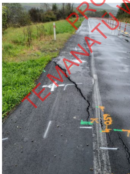
Cracking due to ground movement
