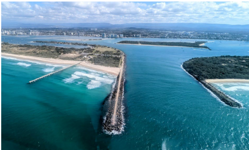
Figure 8.2: Sand bypass system on a jetty structure adjacent to the Gold Coast Seaway (source: Gold Coast Waterways Authority)
